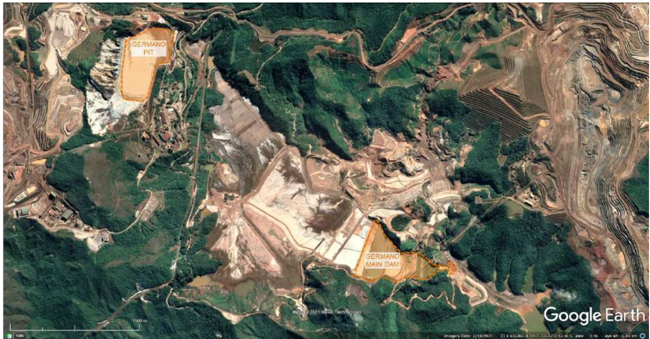
Figure 1. Germaino Main Dam (GMD) and Germaino Pit (GP) structures (Source: Google Earth)
